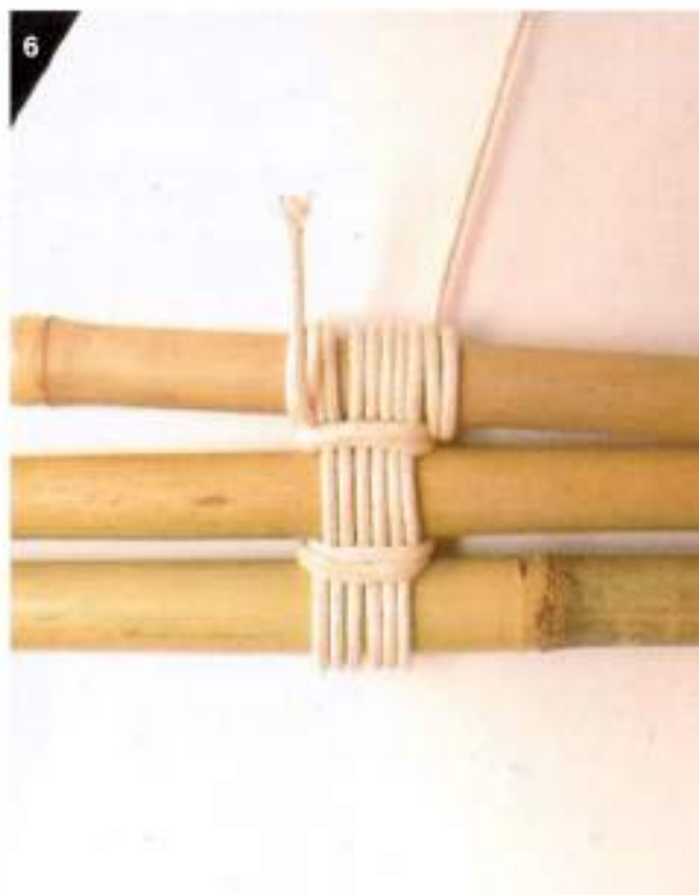
STEP SIX. MAKE A CLOVE HITCH AROUND THE POLE THAT ALREADY HAS A CLOVE HITCH (FROM THE BEGINNING) AT THE OPPOSITE END.
